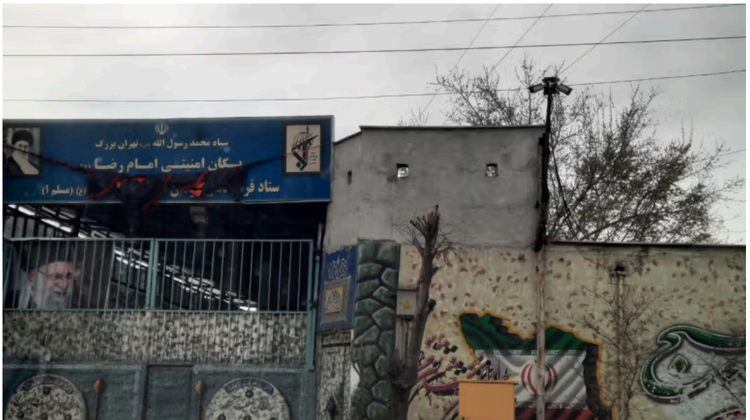
The Imam Reza security unit after sustaining damage, part of the IRGC's Mohammad Rasulullah Corps in Greater Tehran.
